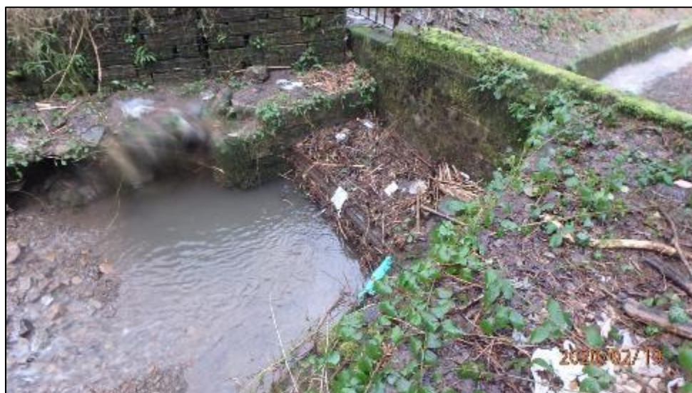
Figure 23: Photo of debris accumulation in the upper reaches of the Nant Coedcaetylleforest ordinary watercourse (below the A4061) (captured by RCT's Flood Risk Management team on 19/02/2020)
